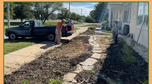
Laying the walkway in Native Pollinator Garden
