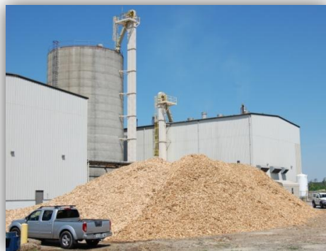
This wood-based 4 MW CHP plant on the Lower Eastern Shore has operated since the 1980s providing heat and electricity to the ECI correctional institution.
