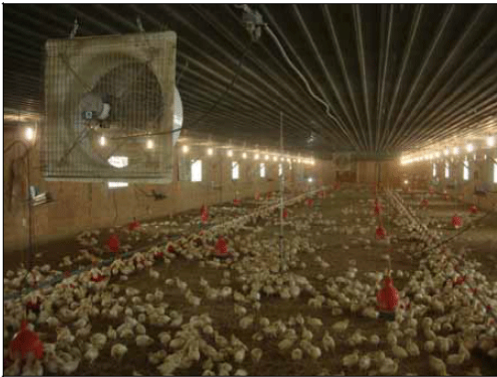
Figure 4. Circulation fan system
