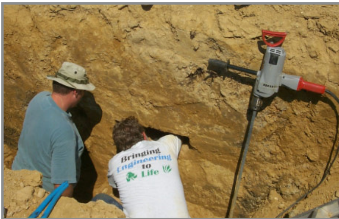
Figure 11. Excavating slot for pan lysimeter installation in granular porous media.
