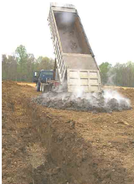
Figure 1. Dumping biosolids next to a prepared trench.
