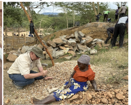
Breaking down rock for dam
