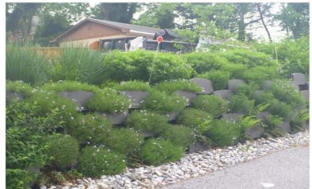
Furbish-designed SmartSlope Vegetated Retaining Wall Photo credit: Carole Barth
