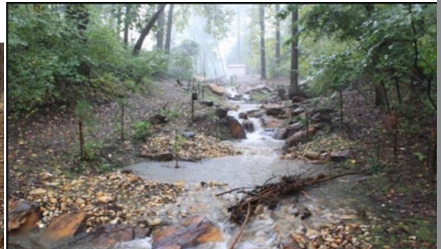
Regenerative Stormwater Conveyance & Riparian Buffer Restoration Credit: Anne Arundel County, MD
