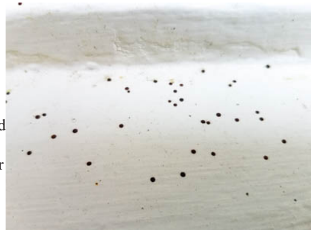
These spots are artillery fungus spores on siding; they can be very difficult to remove Photo: Paul Thomas, Scientific Plant Service
