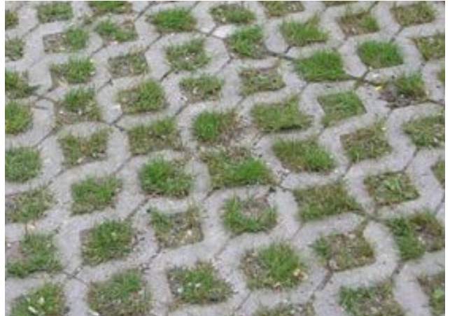
Permeable Pavers. Pavers allow for runoff to filter through the open areas planted with grasses.
