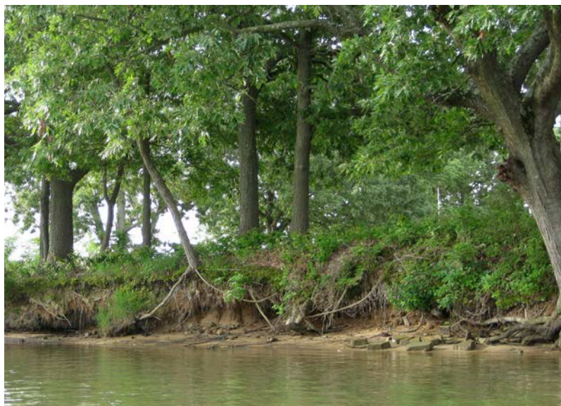
Shoreline Erosion. Trees are undermined by daily tidal action causing them to uproot. When they fall, they carry large amounts of sediment into the creek with them. Photo courtesy of Lisa Marie Ghezzi.
