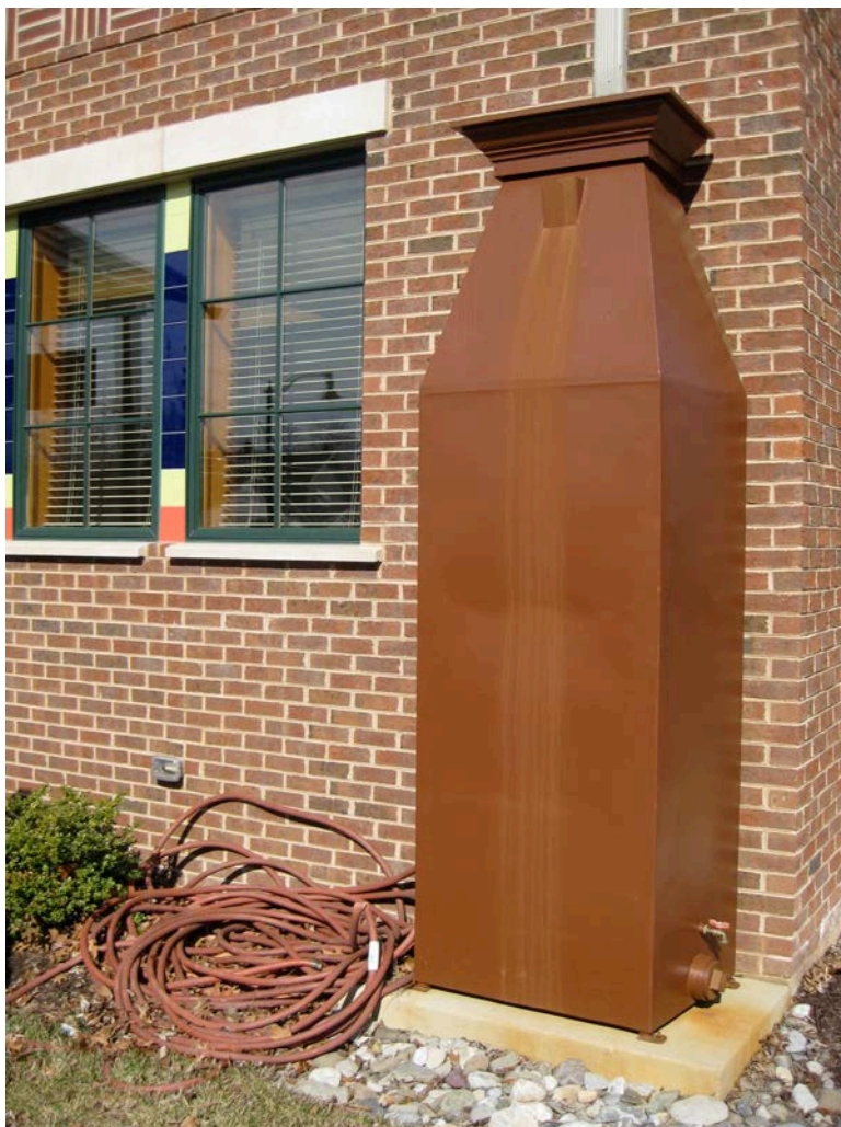
Cistern. This beautiful example of a cistern can be seen if you visit the Talbot County Senior Center, Easton Maryland. Photo courtesy of Lisa Marie Ghezzi.
