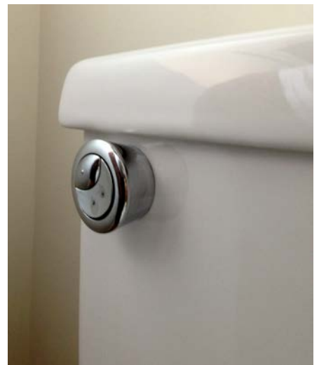
Water Saver Toilet: This inexpensive retrofit can convert any toilet into a water saving toilet.
