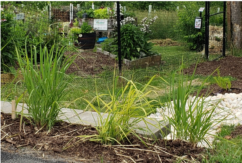
Earlier this summer, the University of Maryland extension offices at 330 Montevue Lane, Frederick, in cooperation with Frederick County government, celebrated a year-long updating and renovation of the storm water management system to a new state-of-the-art system. Shown above are edging grasses and mulch, a part of the filtering system behind the plants, and a portion of the rock drystream bed that will help control and divert water from the parking lot. Stormwater enters into the
