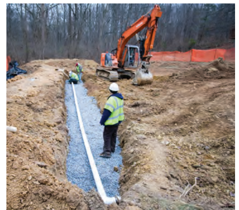
Figure 2.12. Install underdrain on top of initial layer of gravel.
