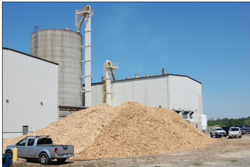
Woodchips outside the ECI CHP facility.
