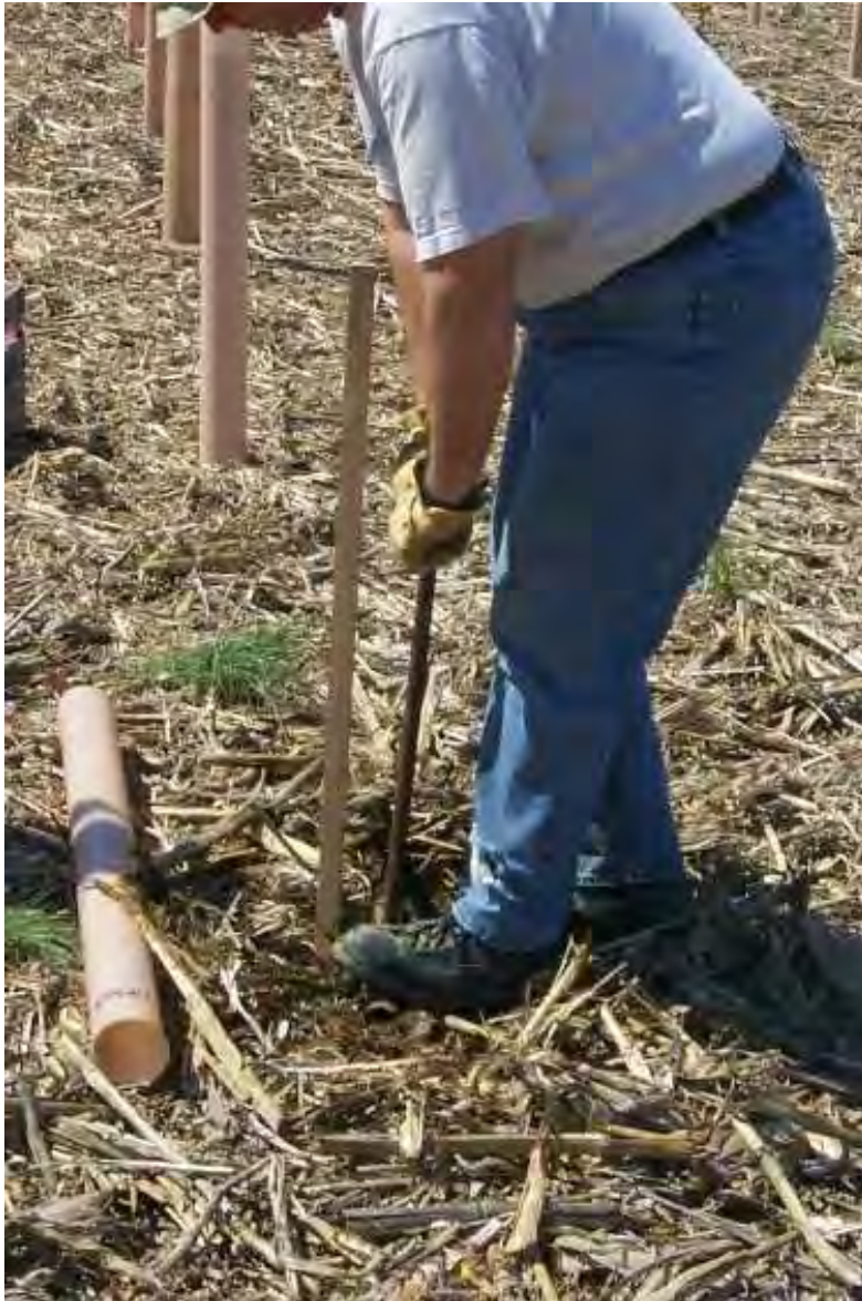
Figure 23. Planting with dibble bar fails to break up compacted soil.
